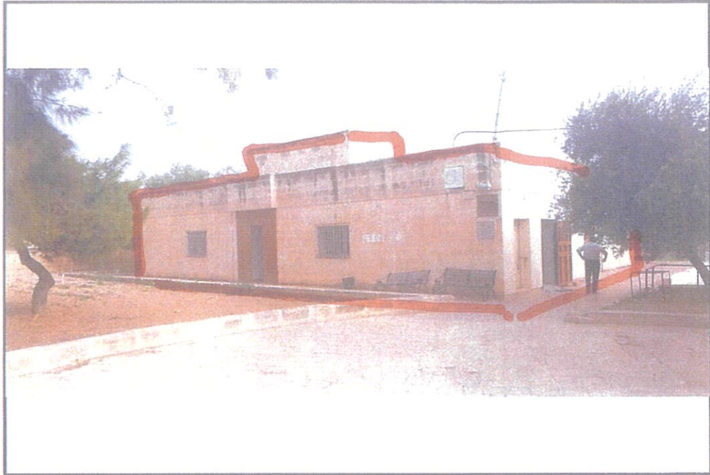
PHOTO No.1--Tribunal Premises main entrance
